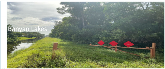
Looking west along the LWDD R/W — existing barricade
