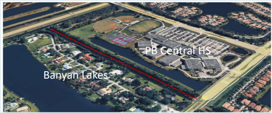
Aerial view southeast toward Palm Beach Central HS
