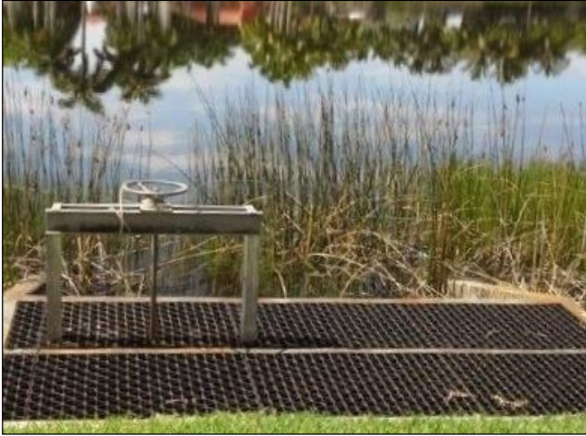
Figure 2: Operable DCS With Above Ground Mechanism
