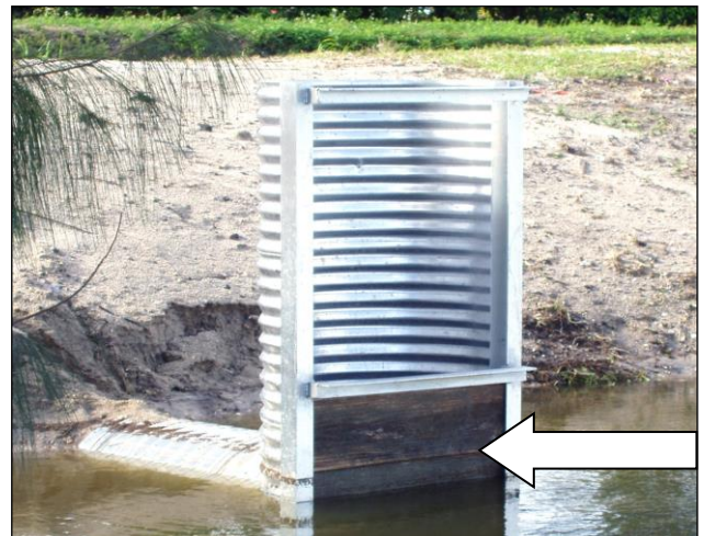
Figure 5: Operable DCS With Wooden Boards
