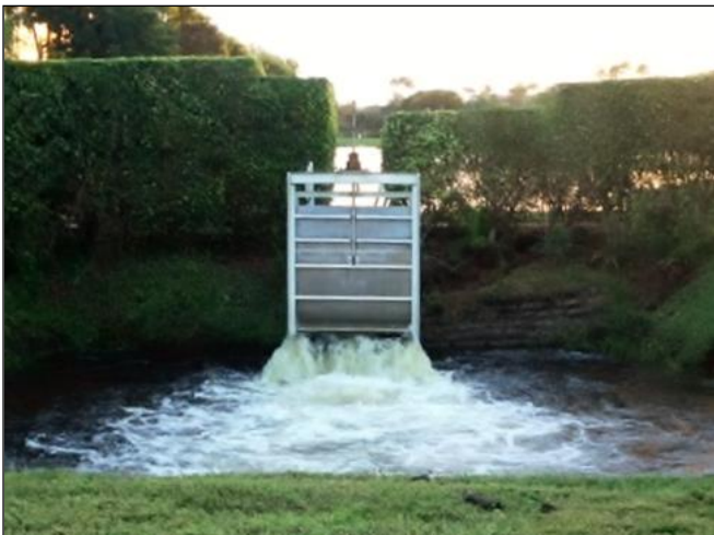
Figure 4: Operable DCS In the Raised/Opened Position
