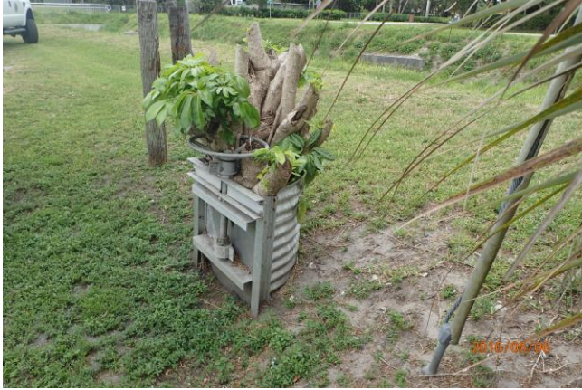
Figure 6: Example vegetation obstructing flow in operable DCS
