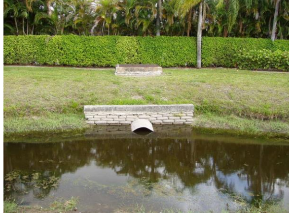
Figure 7: Example of underground connecting pipe to outfall
