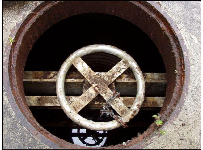
Figure 3: Operable DCS with Below Ground Mechanism
