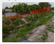
L-14 - Removal of a remaining fence encroachment & vegetation and regrading the low maintenance bank
