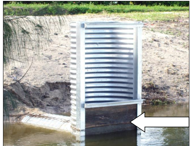
Figure 5: Operable DCS with wooden boards
