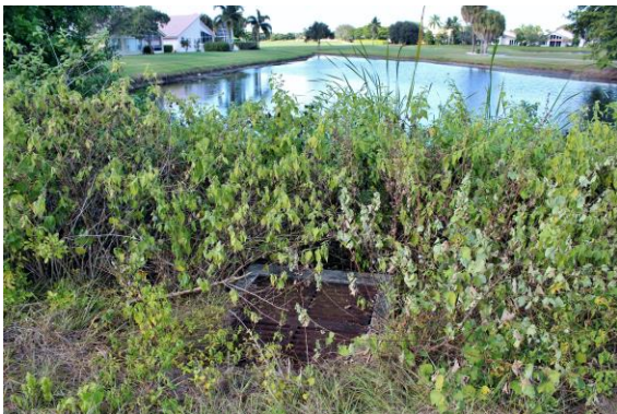
Figure 8: Example of vegetation obstructing flow to catch basins compared to well-maintained catch basin
