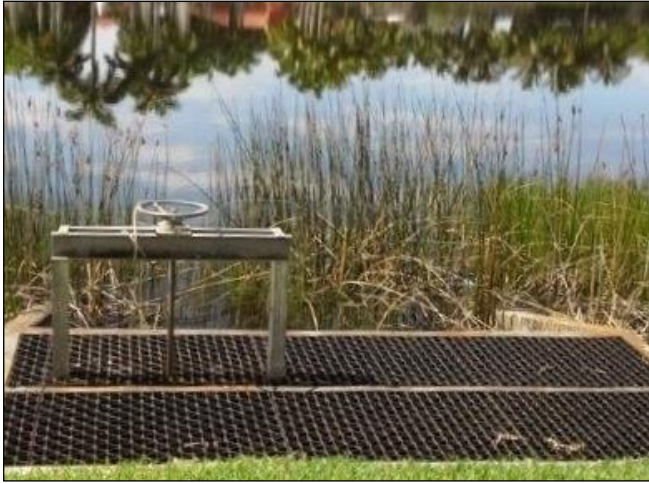
Figure 2: Operable DCS with above ground mechanism
