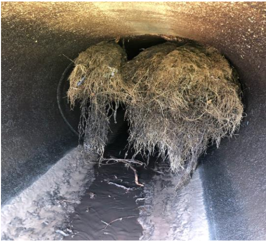
Figure 7: Example of tree roots obstructing flow in pipe compared to well-maintained pipe
