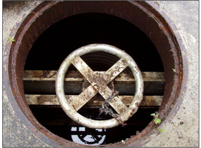
Figure 3: Operable DCS with below ground mechanism
