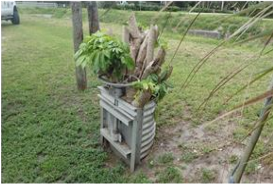
Figure 6: Example of vegetation obstructing water flow in operable DCS compared to well-maintained DCS
