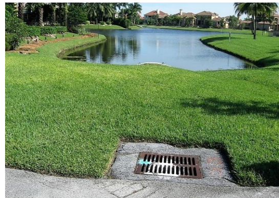
Figure 8: Example of vegetation obstructing flow to catch basins compared to well-maintained catch basin
