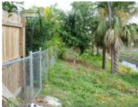
Fence and vegetation located on LWDD right-of-way
