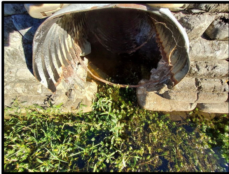
Failing Pipe
