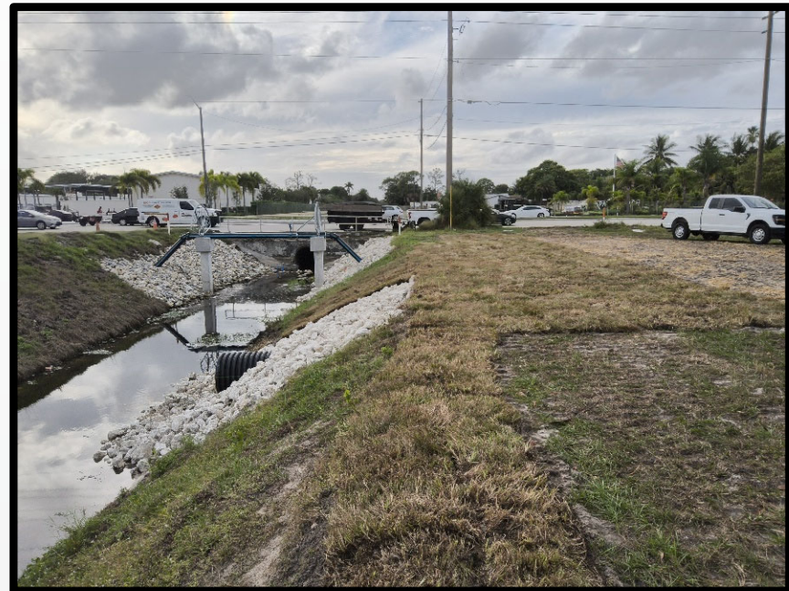
New Outfall Pipe and Restored Bank
